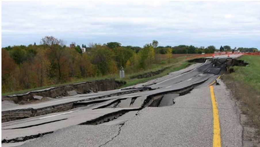
Figure 4. Highway 2 East of Crookston MN, collapsed due to rotational slumping.
